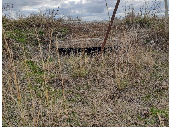
Internal drainage mid -section, southern block – note scouring
